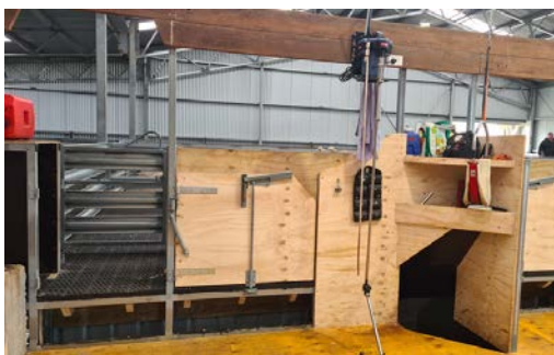
Left: The angle of the catching pen was an important feature of the design. Jarrod noted that the measurements of the race are slightly different to the designs on AWI modules, with the decision made to lower the floor level of the race to make it easier for their shearers to pull the sheep down. Below left: Jarrod King. Below right: Howard Morrison (Morrison Shearing).
