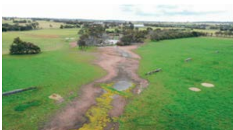
Images below: Before & After Rehabilitation Section 30 September 2021
